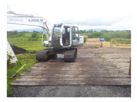
Used as temporary roadways and working platforms, Irish Access Mats' Timber Mats are a simple and effective method of ensuring heavy plant and equipment can traverse soft or boggy terrain without being impeded or causing excessive damage to the land. Our mats are are imported from sawmills in Europe that respect National Forest Management Plans.
